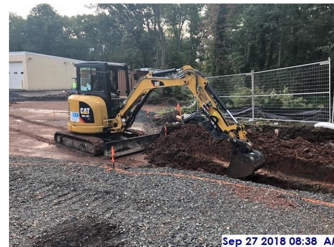
Excavation for new water lines for the new Salt Dome
