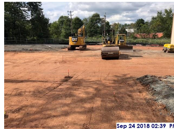
Proof-rolling operations near the new Salt Dome
