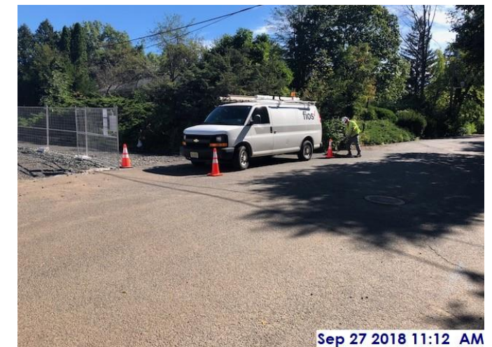
Verizon removing wiring to the Recreation Building.
