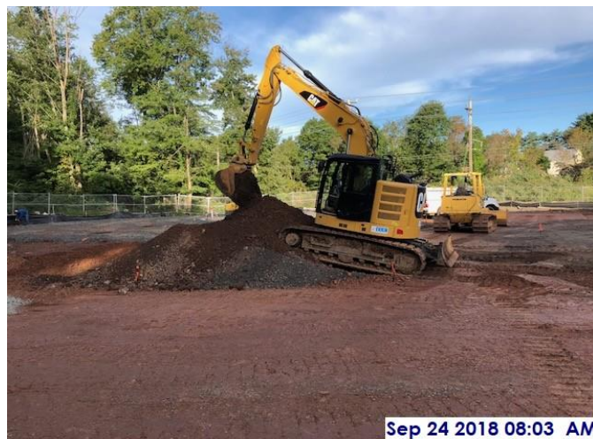
Excavation work near the new Salt Dome
