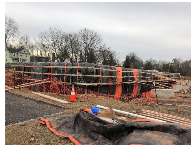
Foundation walls blanketed after concrete pour
