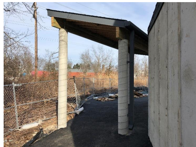
Trim, gutters & downspouts installed at storage shed
