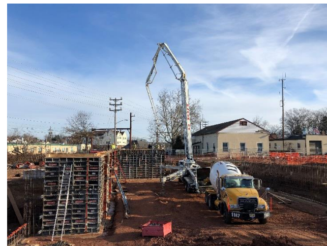
Pumping concrete for foundation walls
